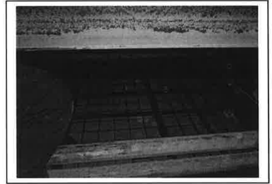
ASH @ TUBES & BEAMS
