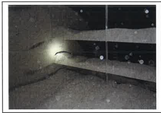
LOWER INLET – EAST SIDE
